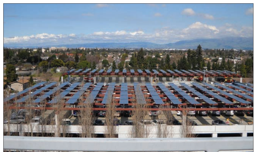
Solar panels already installed on two VMC parking garages will supply 10% of campus-wide energy needs.
